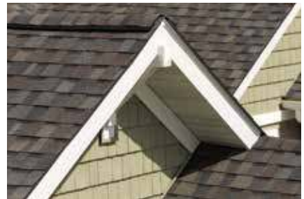
ROOFING AND VENTILATION
